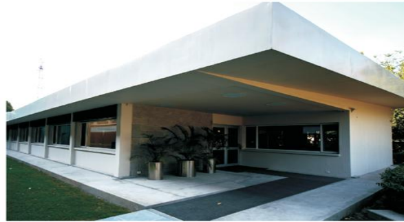
Building made with LC 3 AAC blocks - Swiss Embassy, India
